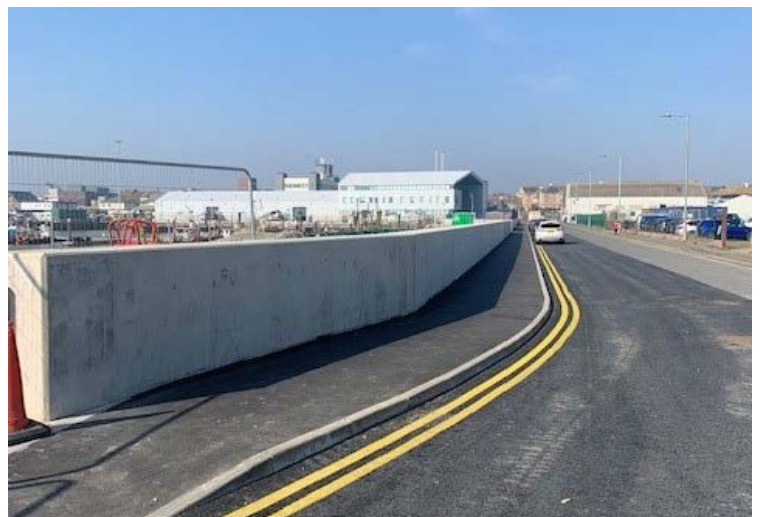
Completed tidal wall on Hamilton Road.
