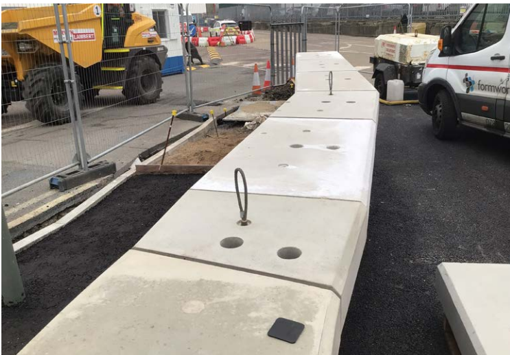
Coping stones near the Port entrance on Waveney Road.
