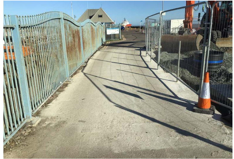
Temporary access to the South Pier.
