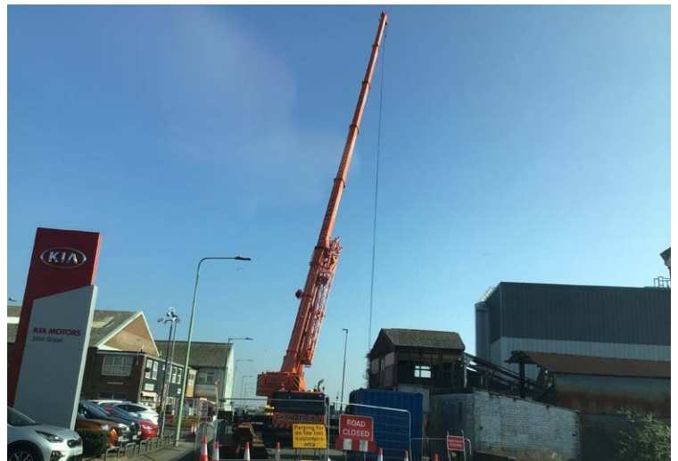
Crane assisting sheet piling works on Hamilton Road.
