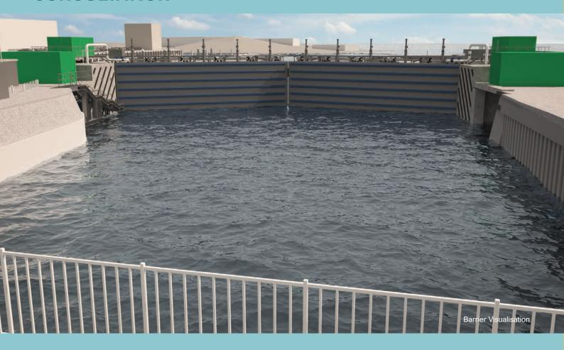
The Lowestoft Tidal Barrier will be built across the channel entrance to Lake Lothing on the seaward side of the Bascule Bridge. Taking the form of a 40m mitre flood gate, the Tidal Barrier will be the second largest of its kind in the UK.
