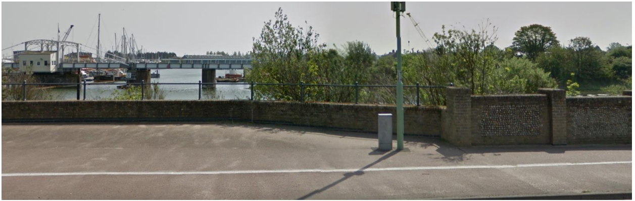
Figure 9 Barrier on the other end of the brick wall © Google 2017
