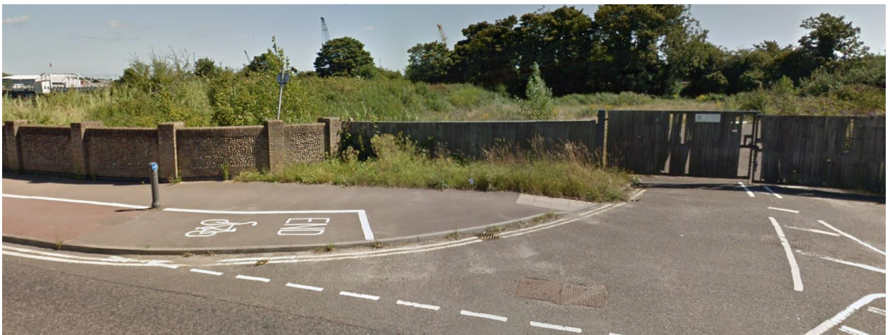
Figure 8 Wooden gate on the end of the brick wall © Google 2017
