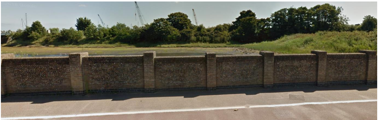
Figure 7 Brick wall on Saltwater Way © Google 2017
